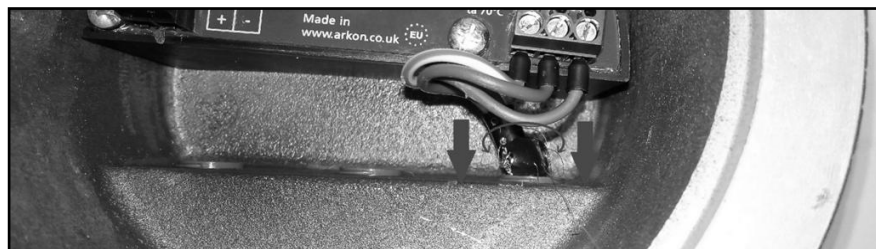
Pic. 3 Manipulation with the cable to achieve sufficient fill up of a cable gland
